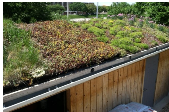
Green rooftop plantings
