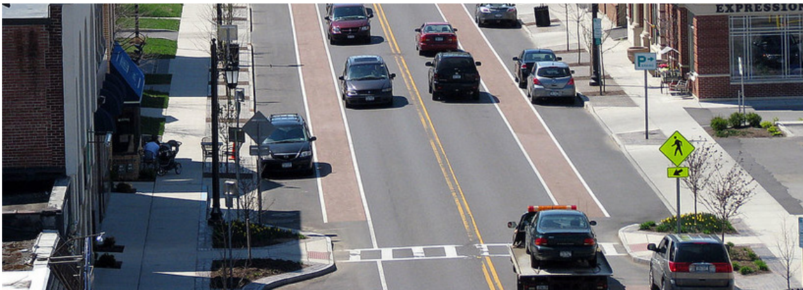
Example of a high-amenity local street with parking on both sides, bicycle paths, sidewalks and pedestrian crossings
