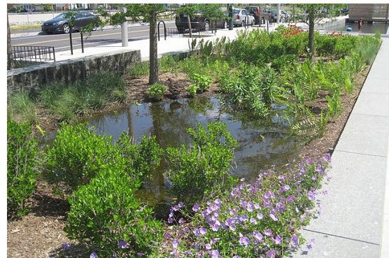
Rain garden/bioretention system
