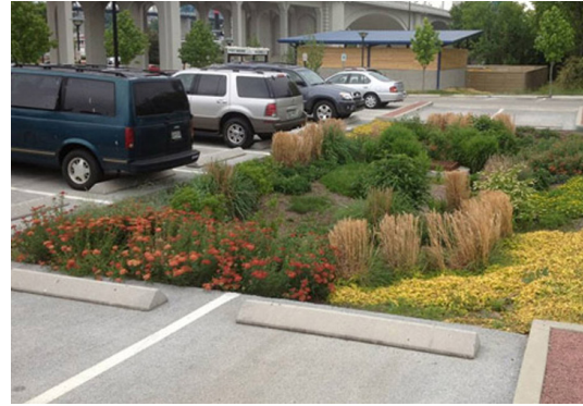
Parking lot stormwater management system with native vegetation
