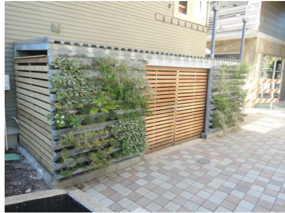
Screening for mechanical equipment and trash receptacles
