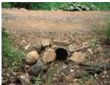
Approaches to culverts crossing drainages should be smooth and level. If the trail narrows or the shoulder is steep, place a warning sign at least 100 feet prior to the hazard.
