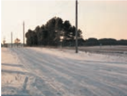
The wide-open sightlines of this trail encourage riders to go faster. The lack of a clearly defined corridor also tempts riders to wander off trail onto adjoining private property, which can lead to trail restrictions. Where the corridor is not obvious, blazes along the trail are recommended to keep riders on the approved trail tread – and remind them of the consequences of not staying on the trail.
