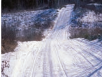
Approaching hills at a right angle is important with snowmobile trails to prevent rollovers. On steep slopes on two-way trails, separating the uphill and downhill sections is sometimes used to increase safety and reduce the potential for conflict. With the open sightlines and modest grade of this hill, two-way traffic on a single 12- to 14-foot tread works well.
