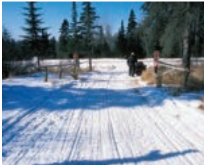
A gateway at this midblock crossing helps snowmobilers and motorists more easily recognize the crossing. The level grade on both sides of the road (similar to a farm field access drive) also improves sightlines and allows the rider to more easily position for the crossing.
