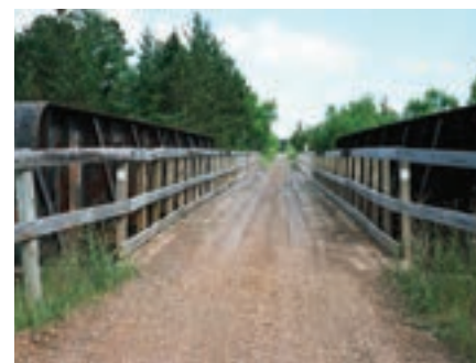
If a summer-use bridge is used for a snowmobile trail, the surface of the trail and deck should be smooth and flush. The deck boards should have minimal gaps to hold snow. Railings are also required.
