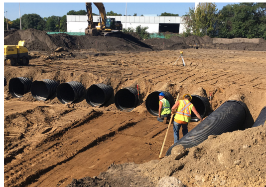
Underground stormwater management
